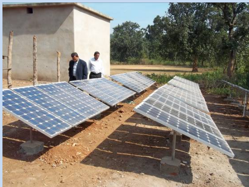
Installation of solar panels under Rural electrification Scheme at Kichinda UPS
