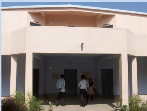
Cyclone shelter in one of the schools in the coastal districts
