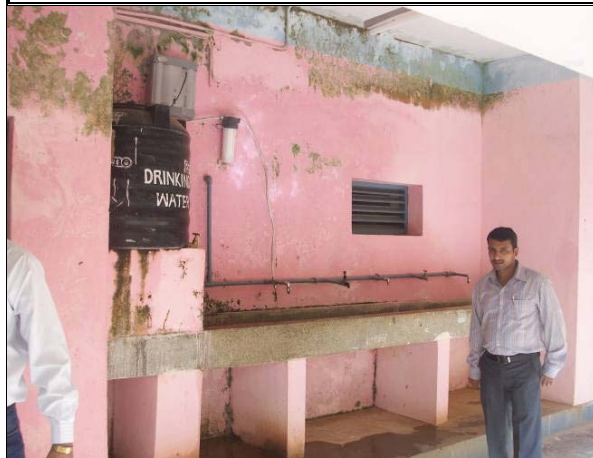
Adequate drinking water taps with a dedicated indoor tank and water treatment facilities at each floor
